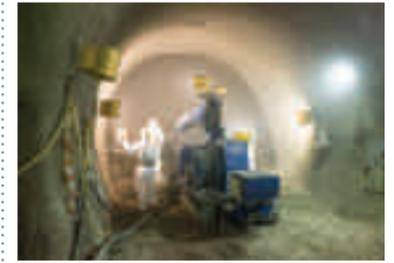
Tunnelling is a major feature of this project, with approximately 300m of sprayed concrete lined tunnels having been constructed in an area where previous tunnelling projects have resulted in ground collapses.
